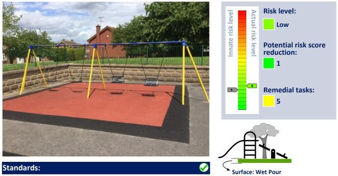
EN 1176-1:2017, EN 1176-2:2017 The item and its surfacing (where applicable) meet with the requirements of the relevant standards.
